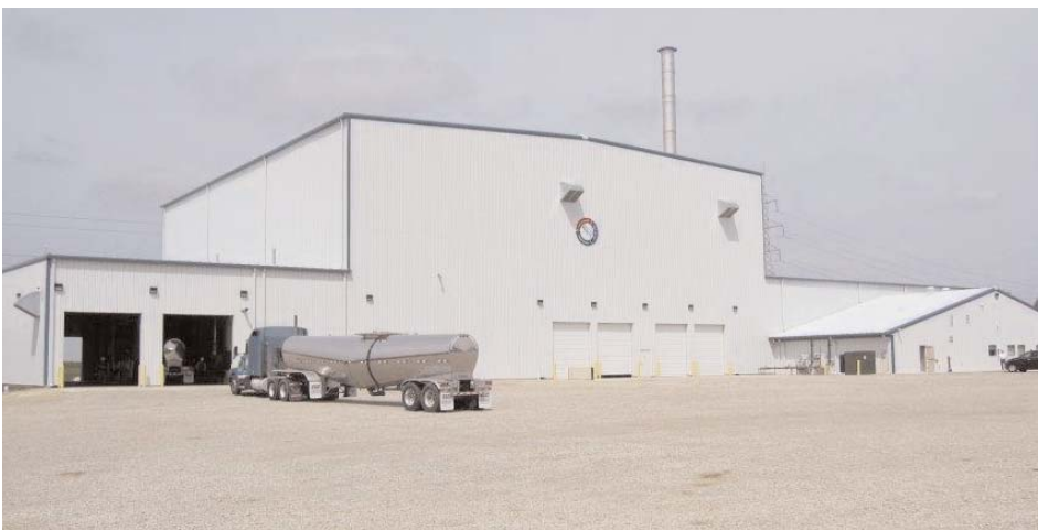
Pictured above: Exterior of NRP-Indiana - 42,000 SF building.
